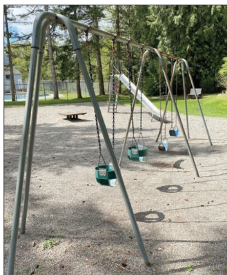
Built in 1990, the much-loved Mays Pond Playground is in need of a long-overdue facelift.
